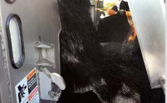
Asphalt can be unloaded incrementally into the paver.
